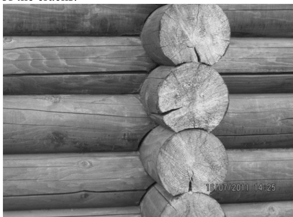
Fig. 1. Surface cracks
